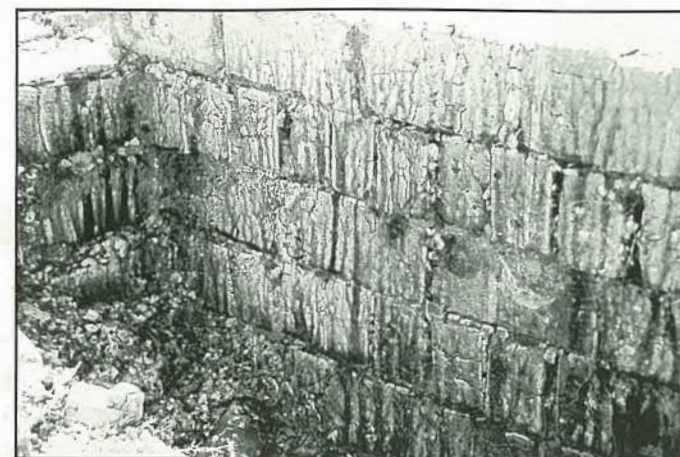
Salt glazed bag wall inside remains of a kiln
