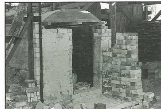
First chamber under construction. The wooden arch-former was used for both chambers. Crusoe starts on the second chamber
