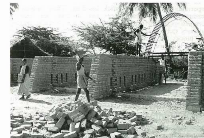
Building the three chambered kiln which will house the watchmen
