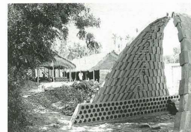
Nubian arch being made with extruded hollow bricks
