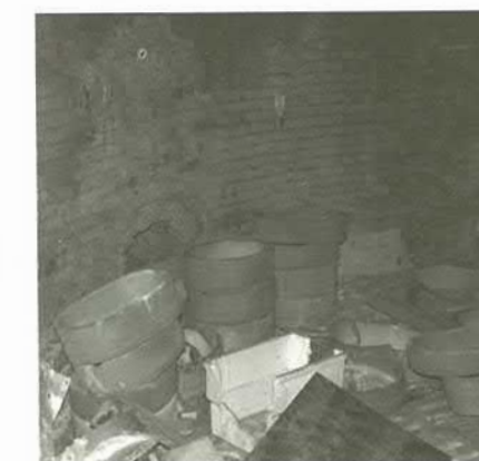
Inside a kiln showing fireboxes and the low continuous bagwall — plus some saggars.
