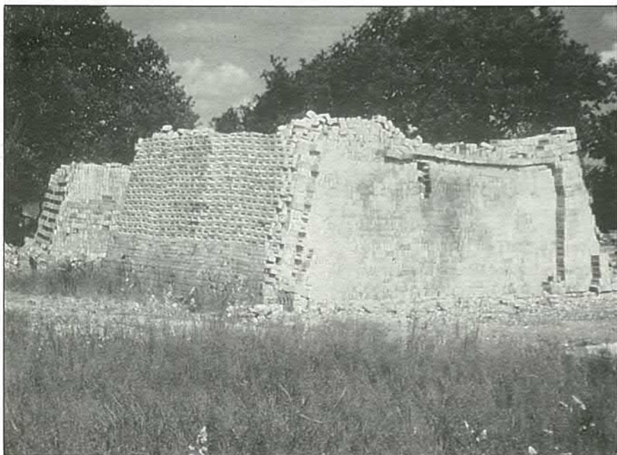
Partially dismantled fired clamp
