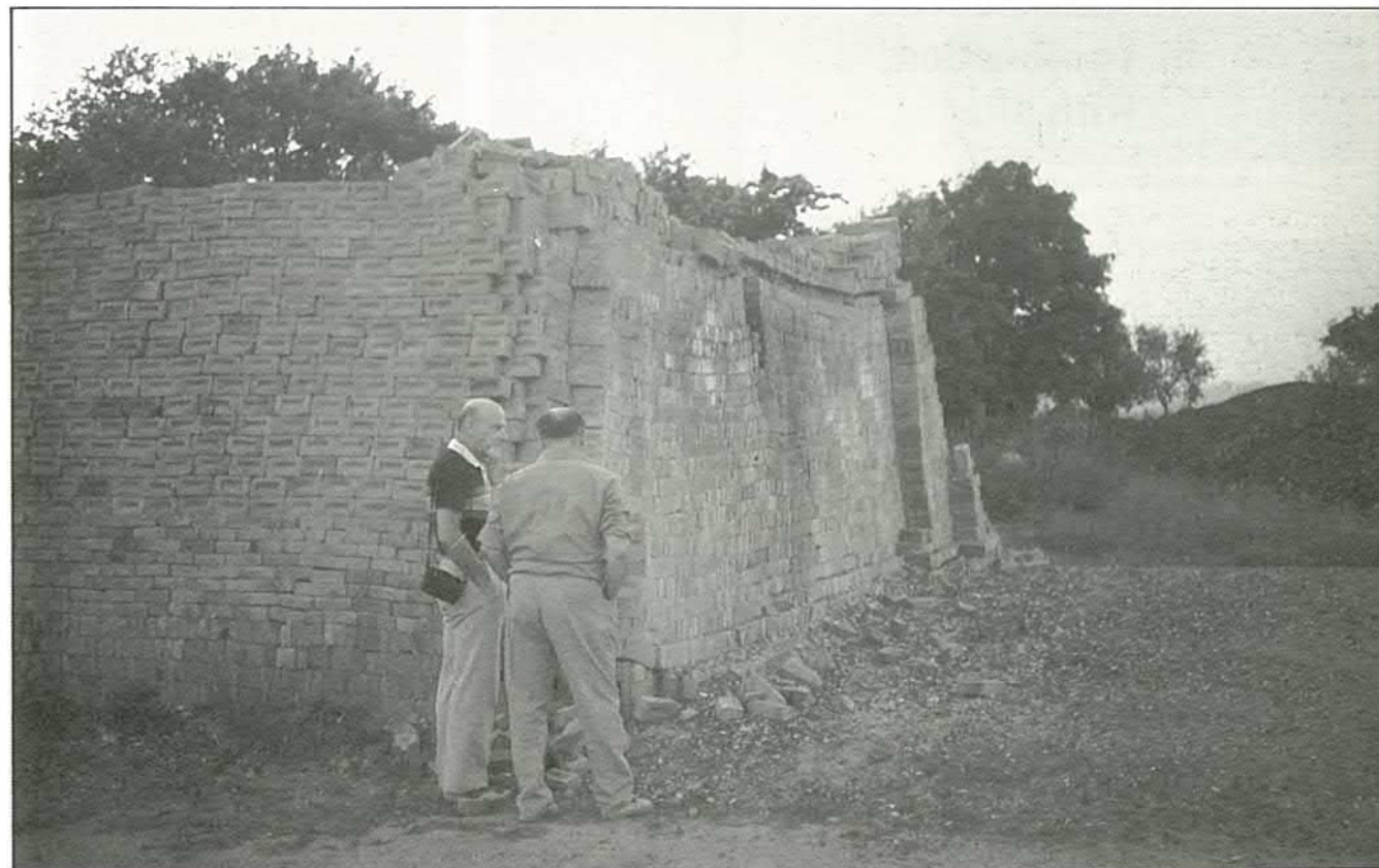
Leo King, left, with Noel Pyecroft at the clamp. The case of burnovers is easily visible
