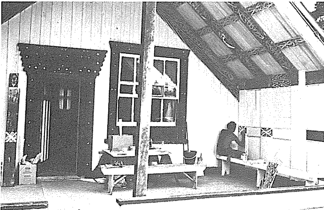
Work in progress in the porch — note some of the poor overpaints on the rafters.
