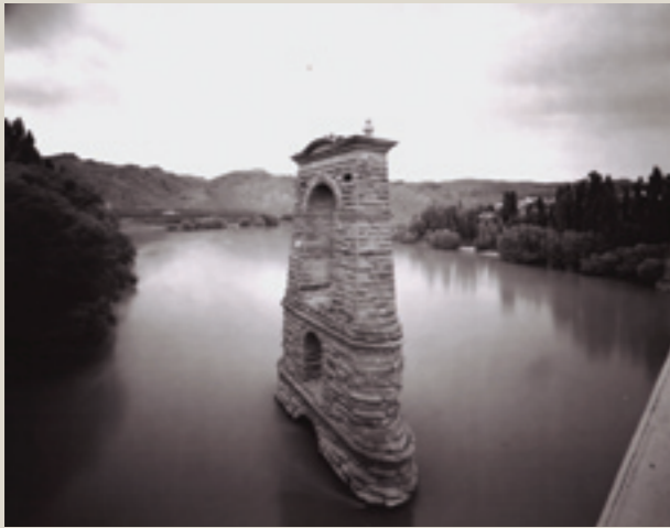
Old bridge structure from new bridge, Clutha River, Alexandra, December 1980
