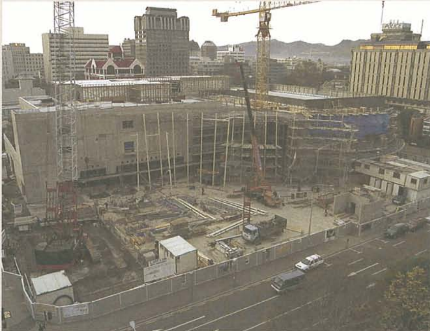
Above: Aerial photograph of the construction of the new Christchurch Art Gallery. Photograph Skyworks Canterbury.
