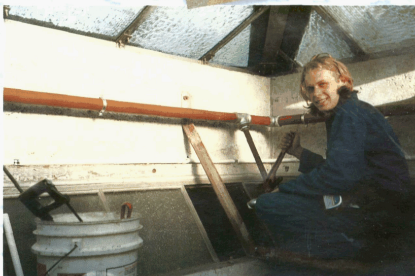
Installing the sprinkler system
