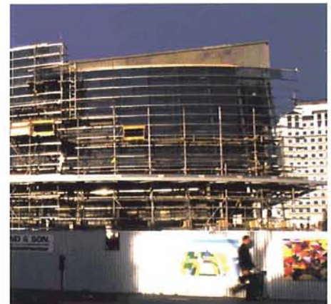
Below: The glass sculpture wall still under construction.
